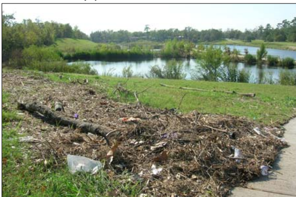
Mason Park Treatment Wetland survived significant storm surge from Hurricane Ike, a category 2 storm with category 4 storm surge (Notice the trash line in the foreground).
